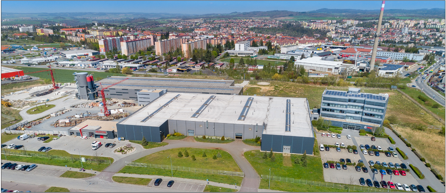
Company's headquarters and production halls
