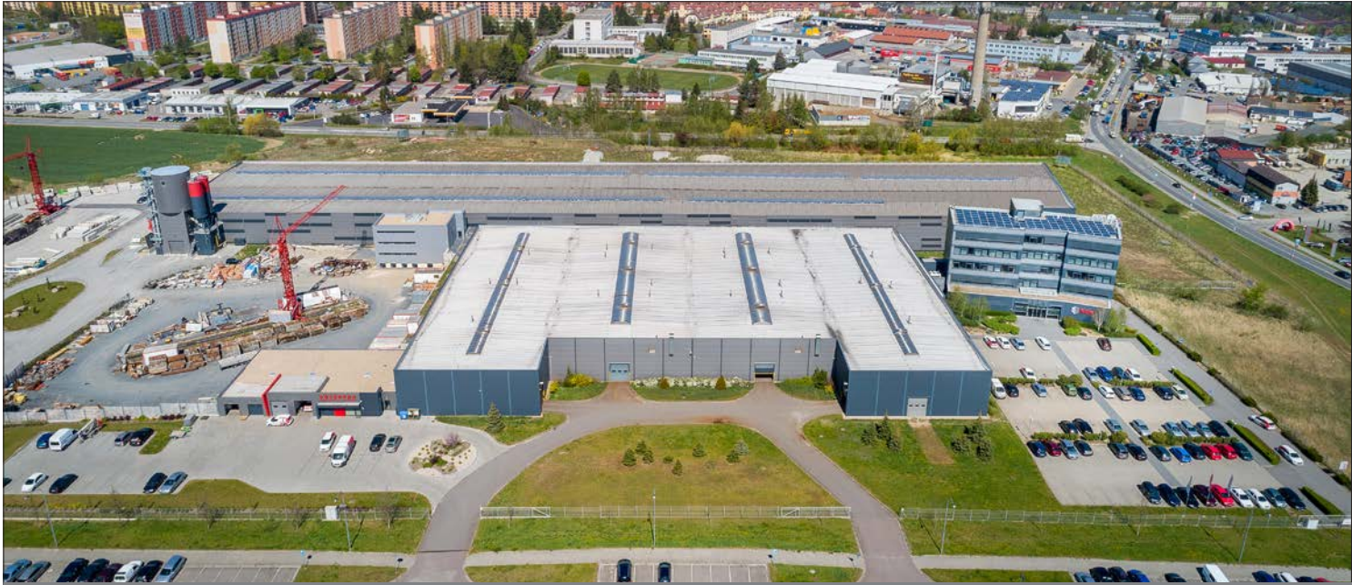
Company's headquarters and production halls
